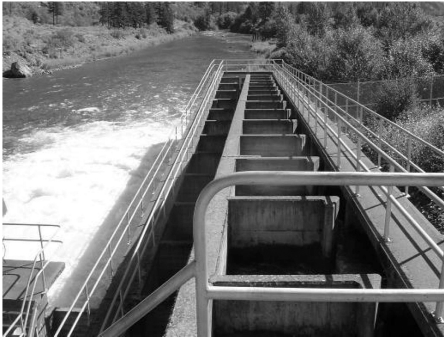
Fig. 1. Vertical slot fishway at the Seton river hydropower facility used to facilitate upstream migration of salmonids (photo source, L.B. Pon).
